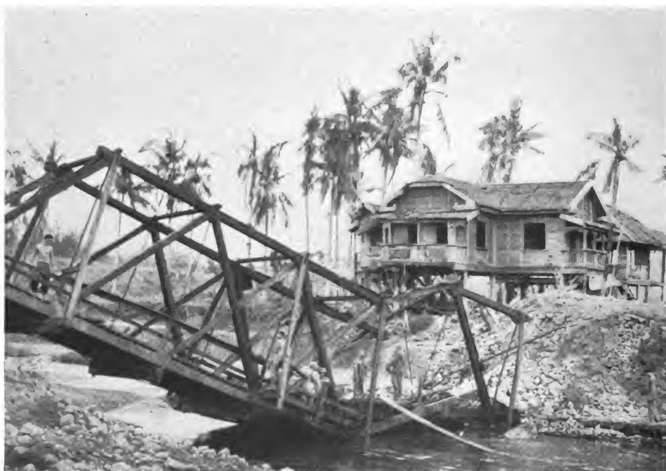
Top: The muddy roads inside Ormoc present almost as troublesome an obstacle as the Jap. Bottom: One of the many bridges knocked out by the U. S. Army Air Forces. Another job for the Engineers!
